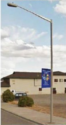
EXISTING STREET LIGHT With banner
