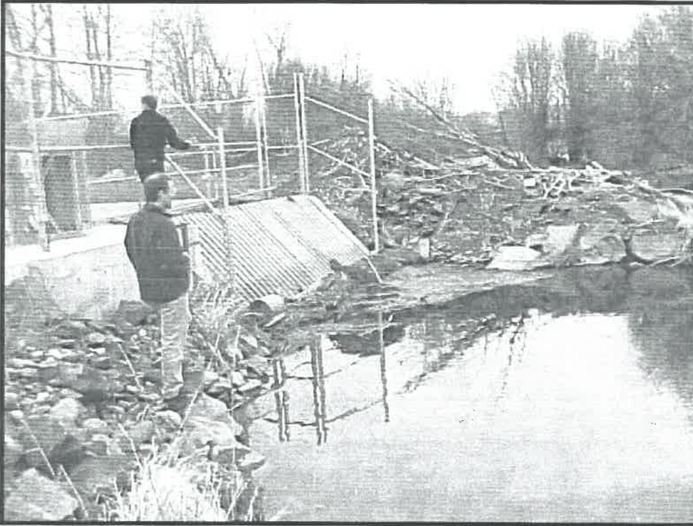
Mill Ditch Diversion intake structure (looking downstream)
