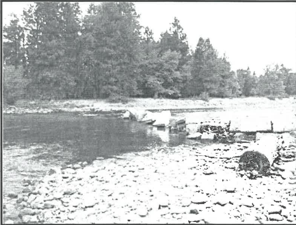
View looking at ecology block dam in Yakima River from upstream (10/31/2001)
