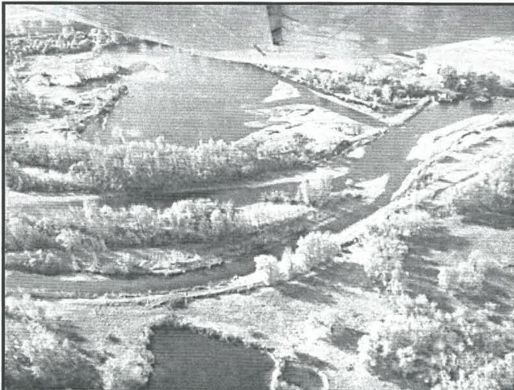
Aerial View of Packwood-Gladmar-Cascade Flow split looking south
