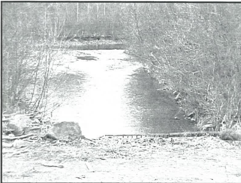
Mill Ditch Diversion Channel Split from Side Channel of Yakima River (looking west)
