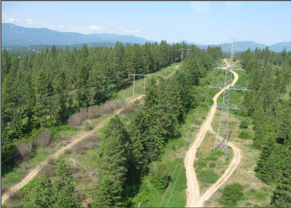
Photograph: Power lines
