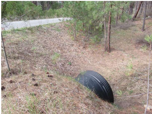
Photo 2 – Facing northeast. East of Summit View Drive. Runoff flows into 48" HDPE culvert
