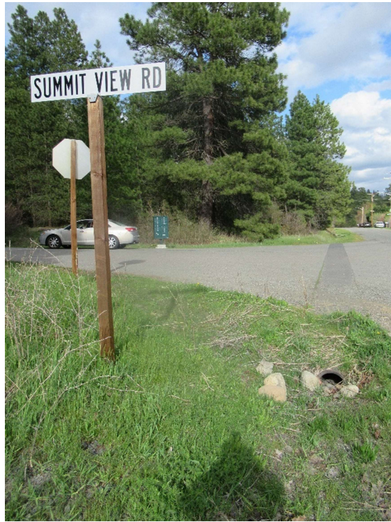
Photo 3 – Facing north. 18 RCP" culvert crossing 6 th St.
