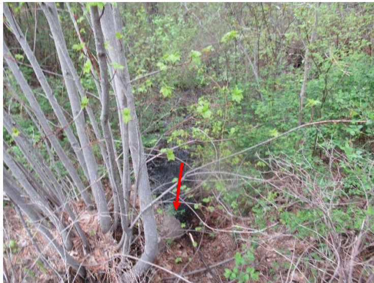
Photo 4 – Facing north. 18 RCP" culvert crossing 6 th St.
