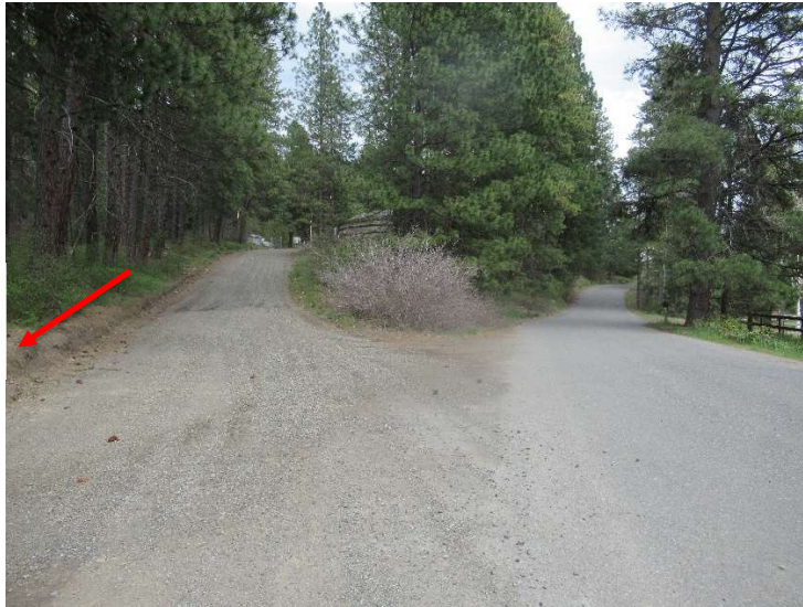
Photo 1 – Facing east. Runoff sheet flows west towards culvert under 6 th St.
