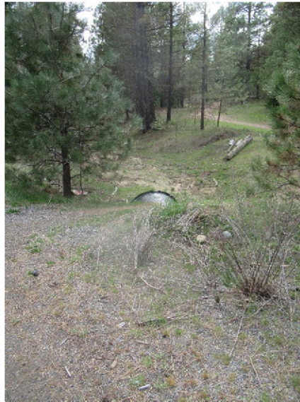
Photo 3 – Facing southwest. West of Summit View Drive. Runoff flows out of 48" HDPE culvert (Crystal Creek 3 Basin 3).
