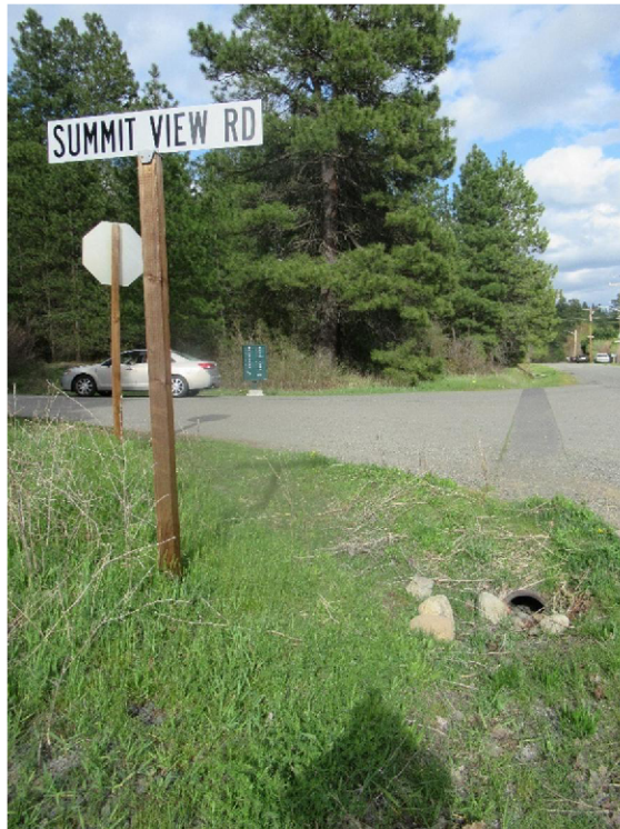
Photo 3 – Facing north. 18 RCP" culvert crossing 6 th St.
