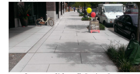
Concrete Sidewalk Paving Pattern
