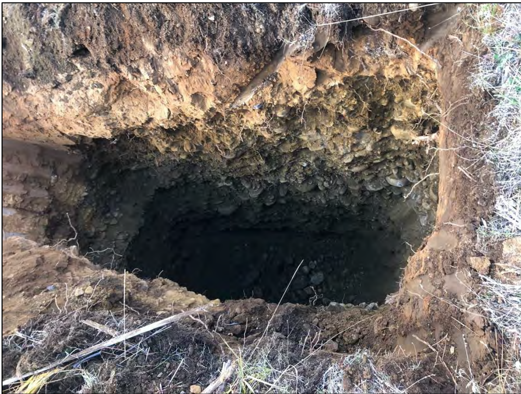
Figure 4. Representative photograph of the subsurface conditions observed in EP-28.
