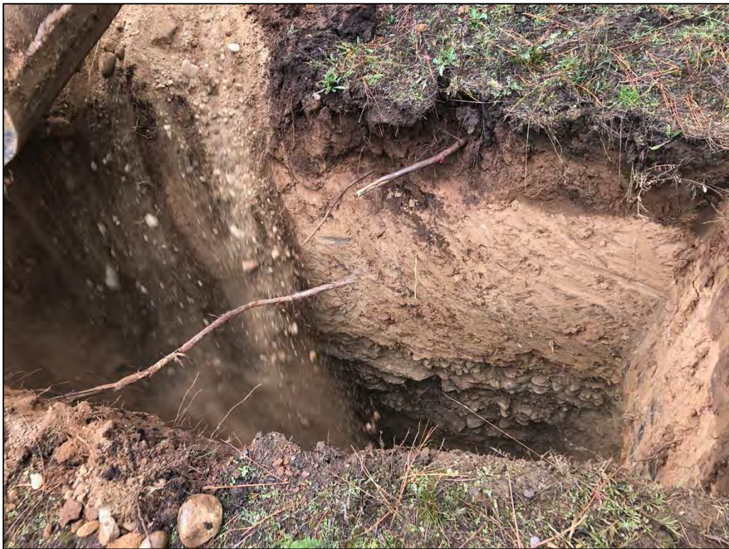
Figure 4. Representative photograph of the subsurface conditions observed in EP-4.
