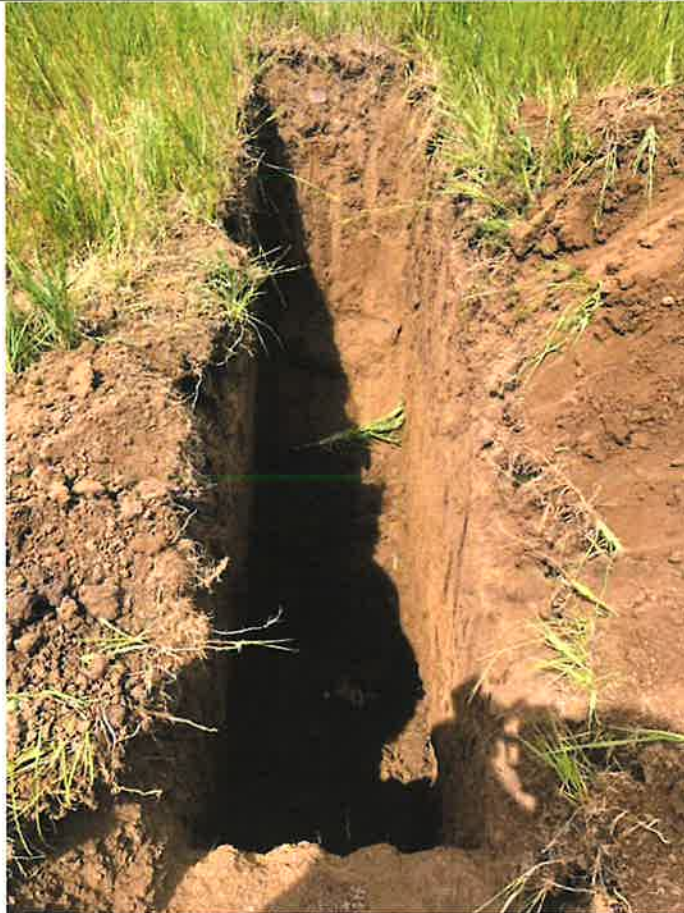
Completed test pit.
