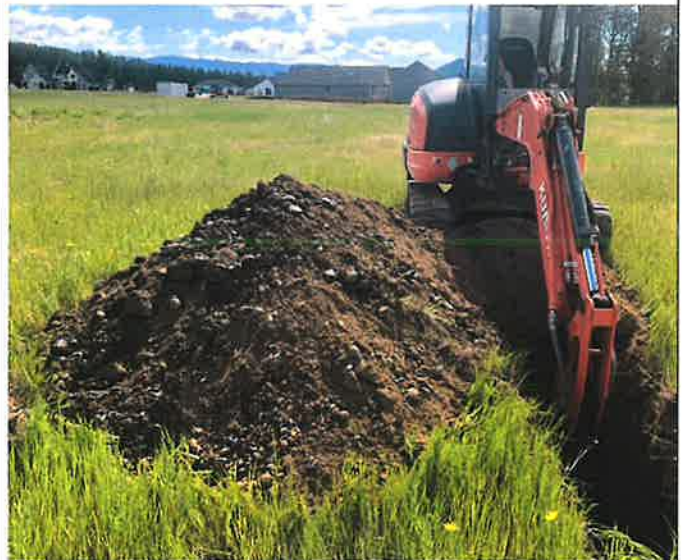
Test pit spoils.
