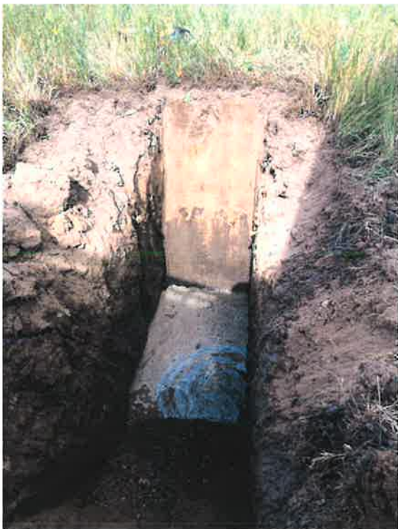
Completed test pit.
