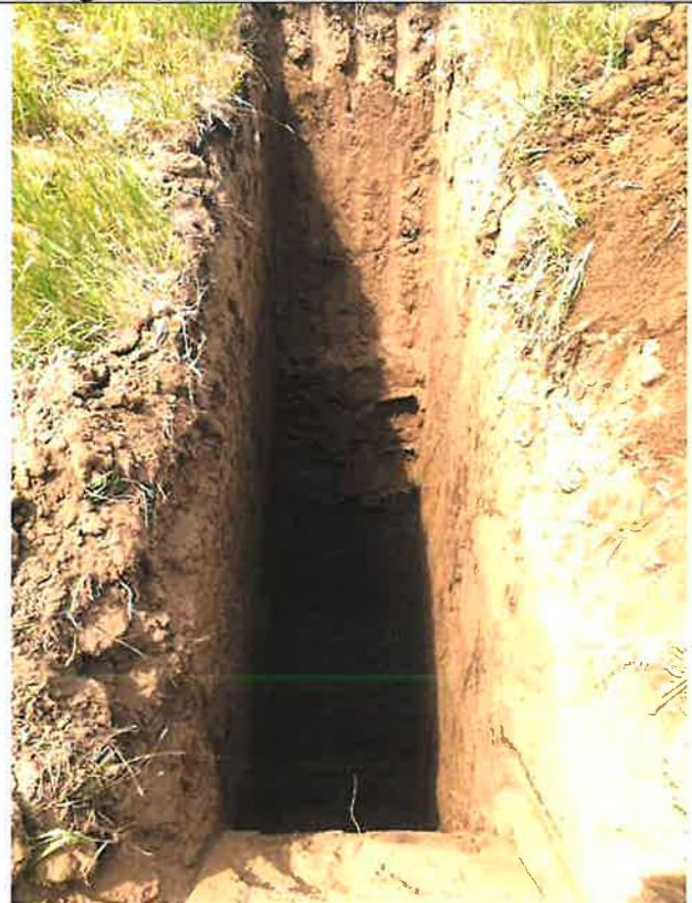
Completed test pit.
