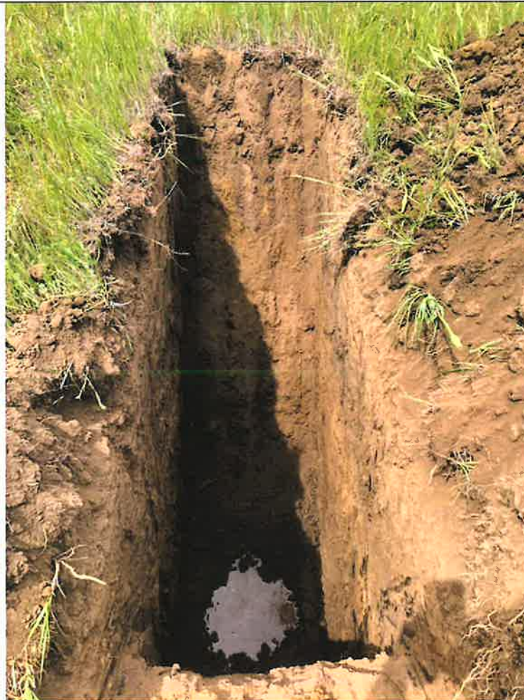
Completed test pit.
